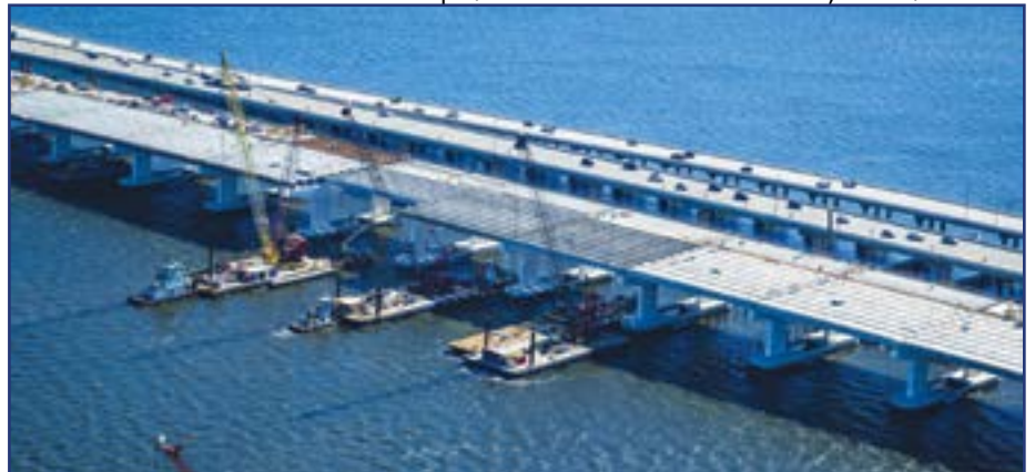
Construction of New Span, January 2025 Credit: FDOT
