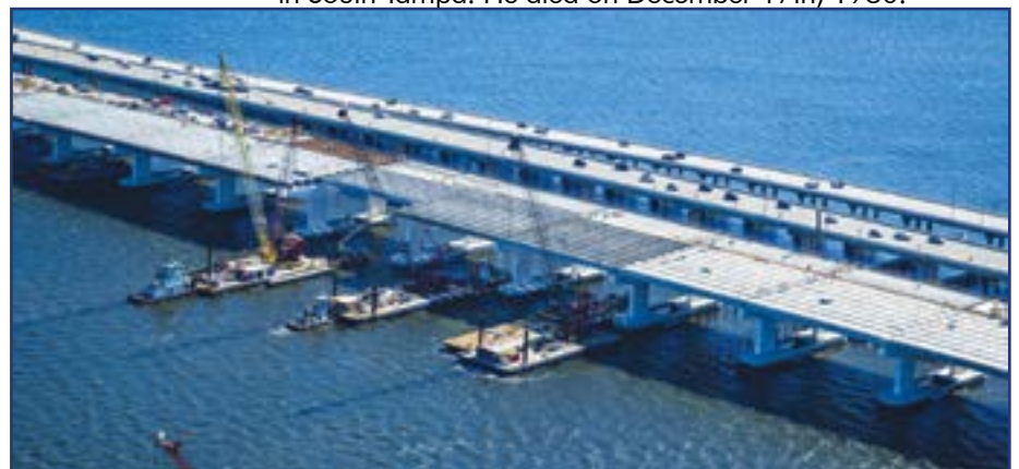
Construction of New Span, January 2025 Credit: FDOT
