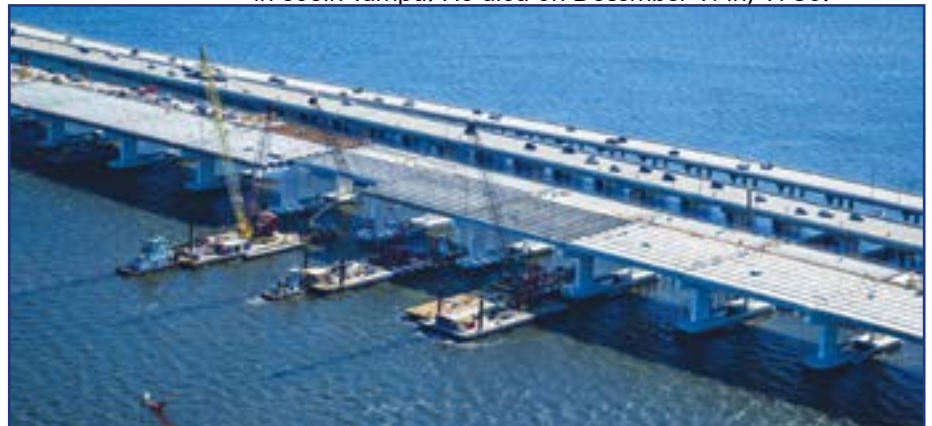
Construction of New Span, January 2025 Credit: FDOT
