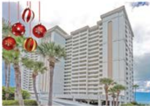
LANDMARK TOWERS I - SAND KEY 1230 Gulf Blvd #304 1BR | 1.5BA | 869sf | $625,000
