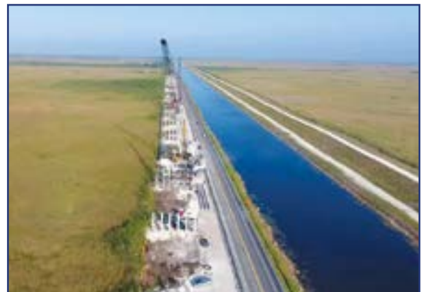
Tamiami Trail Next Steps Construction
