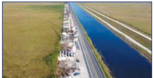
Tamiami Trail Next Steps Construction
