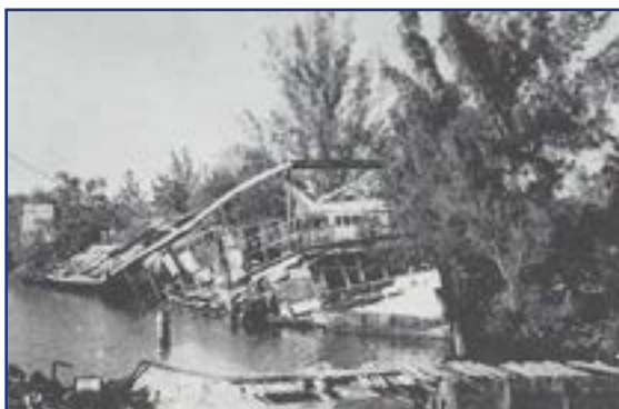
The Nushka in dilapidated condition
