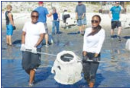
Concrete Oyster Reef Ball installation
