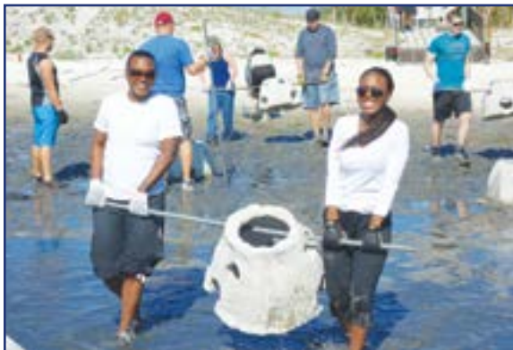
Concrete Oyster Reef Ball installation
