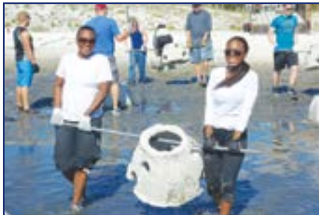
Concrete Oyster Reef Ball installation
