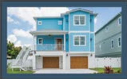
New Home Construction
