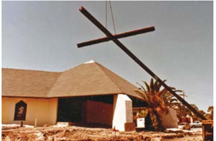
1960 - Construction of the first church on Hamlin Blvd.
